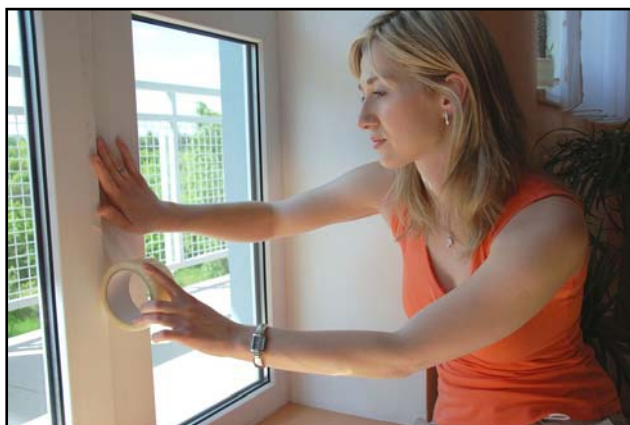
Fig.: Sealing windows with a tape
