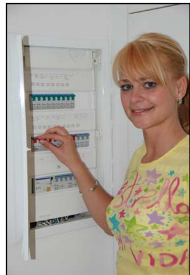
Fig.: turning off the main electric circuit breaker
